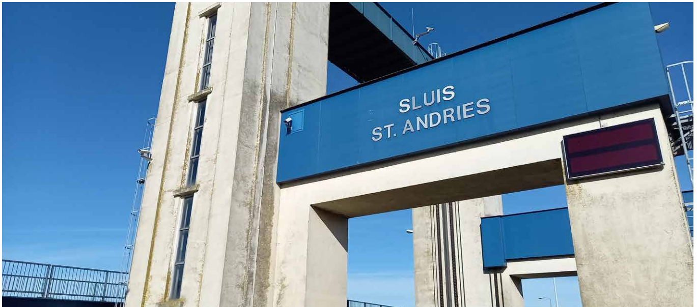
Sluis Complex St. Andries
